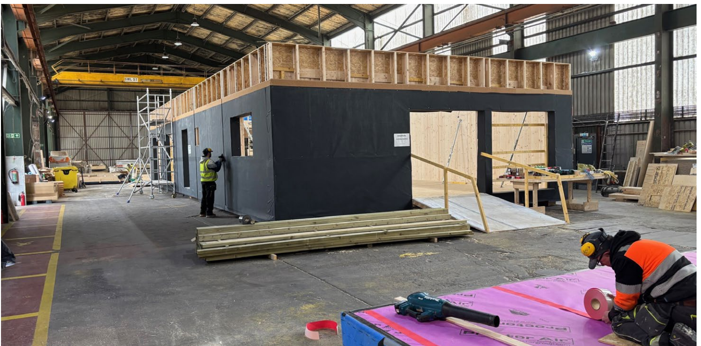
A community hub under construction in the Ecosystems Technologies factory
