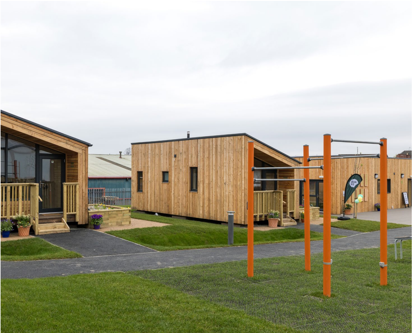
Greenery, plants and an outdoor gym space at the Social Bite Village in Rutherglen, South Lanarkshire
